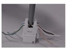
c) Trim the wires flush with the IDC towers.
