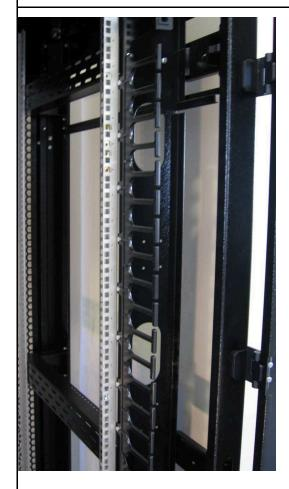
4.2) Fasten the 19" Vertical Rack Manager to a Cabinet using 6 Philips type screw
