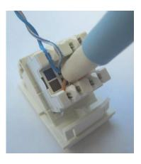
**c) Cable strain relief:** Fit cable strain relief stuffer cap ensuring the "U" shape cut-out follows the direction of the incoming cable.
