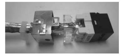
6j. Ensure cables are trimmed off flush with IDC, if not use side cutters to remove excess cable after termination.
