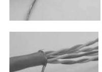
4c. Remove foil from pairs of cable. Twist braid and wrap around the cable sheath
