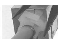
6c. Remove 3 of the 4 foils from the cable pairs. Unwrap the foil from 1 pair in preparation for Wrapping around the cable sheath.
